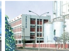
DTY Plant III 1997
