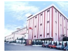
DTY Plant I 1969
